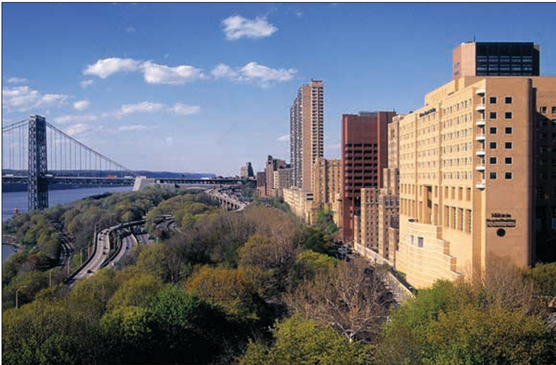
NewYork-Presbyterian/Columbia University Irving Medical Center on New York City's Riverside Drive
