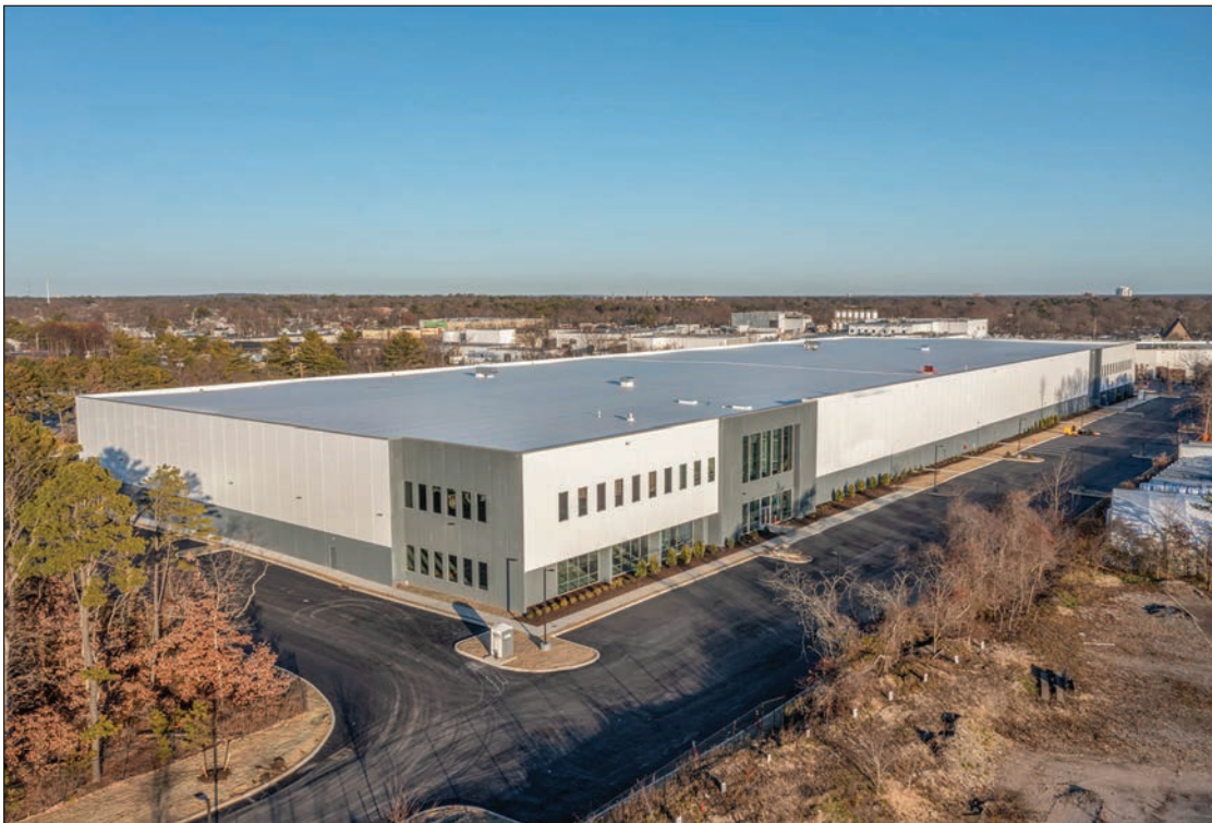
The newly completed 55 Paradise Lane, Rockefeller Group's 172,622-square-foot distribution center on approximately 11 acres in Bayside, New York
