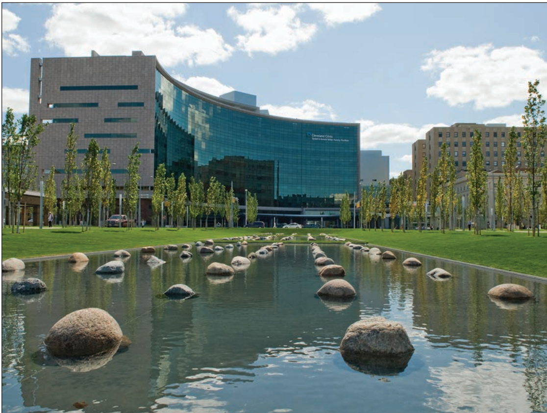
Miller Pavilion at Cleveland Clinic's main campus in Cleveland, Ohio (above and below)
