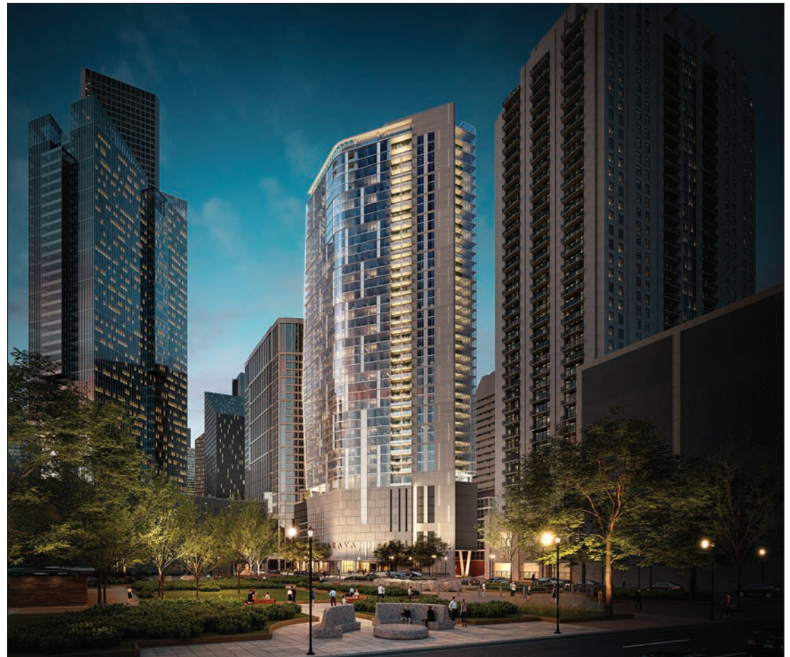
Hines, along with Cresset Wealth Advisors and Levy Family Partners, are developing Brava, a luxury for-rent residential high-rise community in Houston
