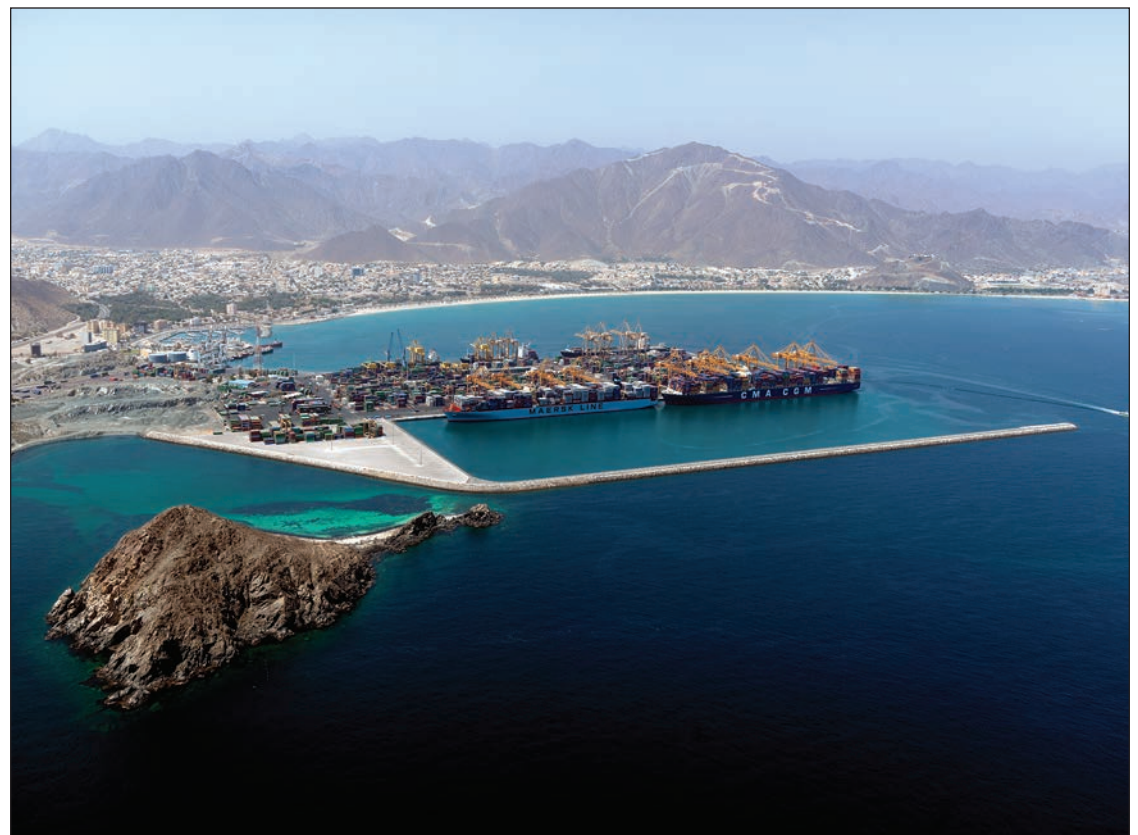
Gulfstainer, Khorfakkan Container Terminal
