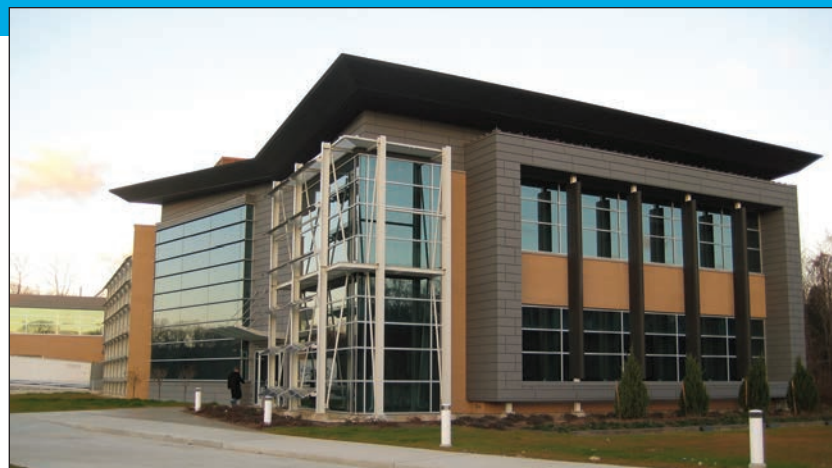
Advanced Energy Research and Technology Center at Stony Brook University
