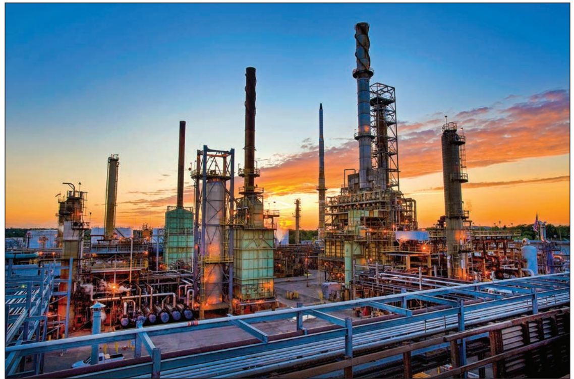
Marathon Petroleum Corp.'s refinery in Canton, Ohio, is part of the corporation's seven-refinery system, which can process approximately 1.8 million barrels per day of crude oil (above); Marathon Petroleum Corp. owns, leases, or has an ownership interest in 10,800 miles of crude oil and light product pipelines and more than 5,600 miles of gas gathering and natural gas liquids pipelines (below)
