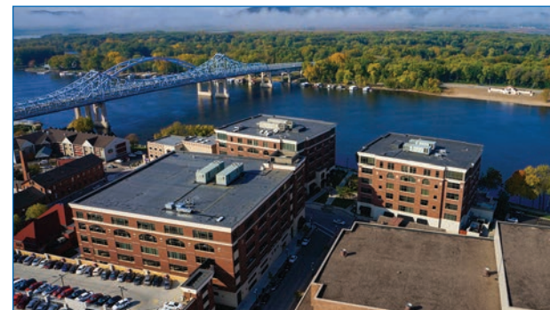
Logistics Health Incorporated's headquarters in La Crosse, Wisconsin
