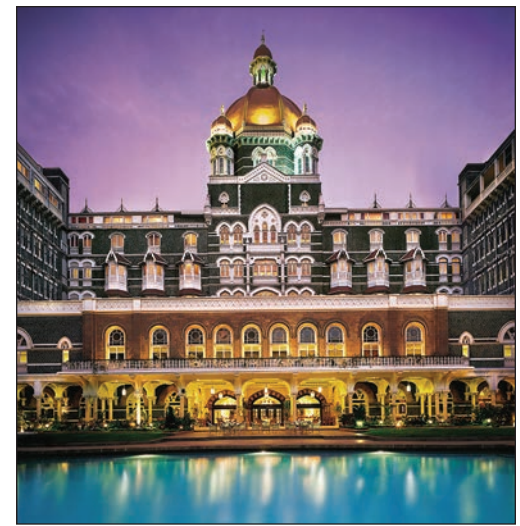
The iconic dome and pool of The Taj Mahal Palace, Mumbai
