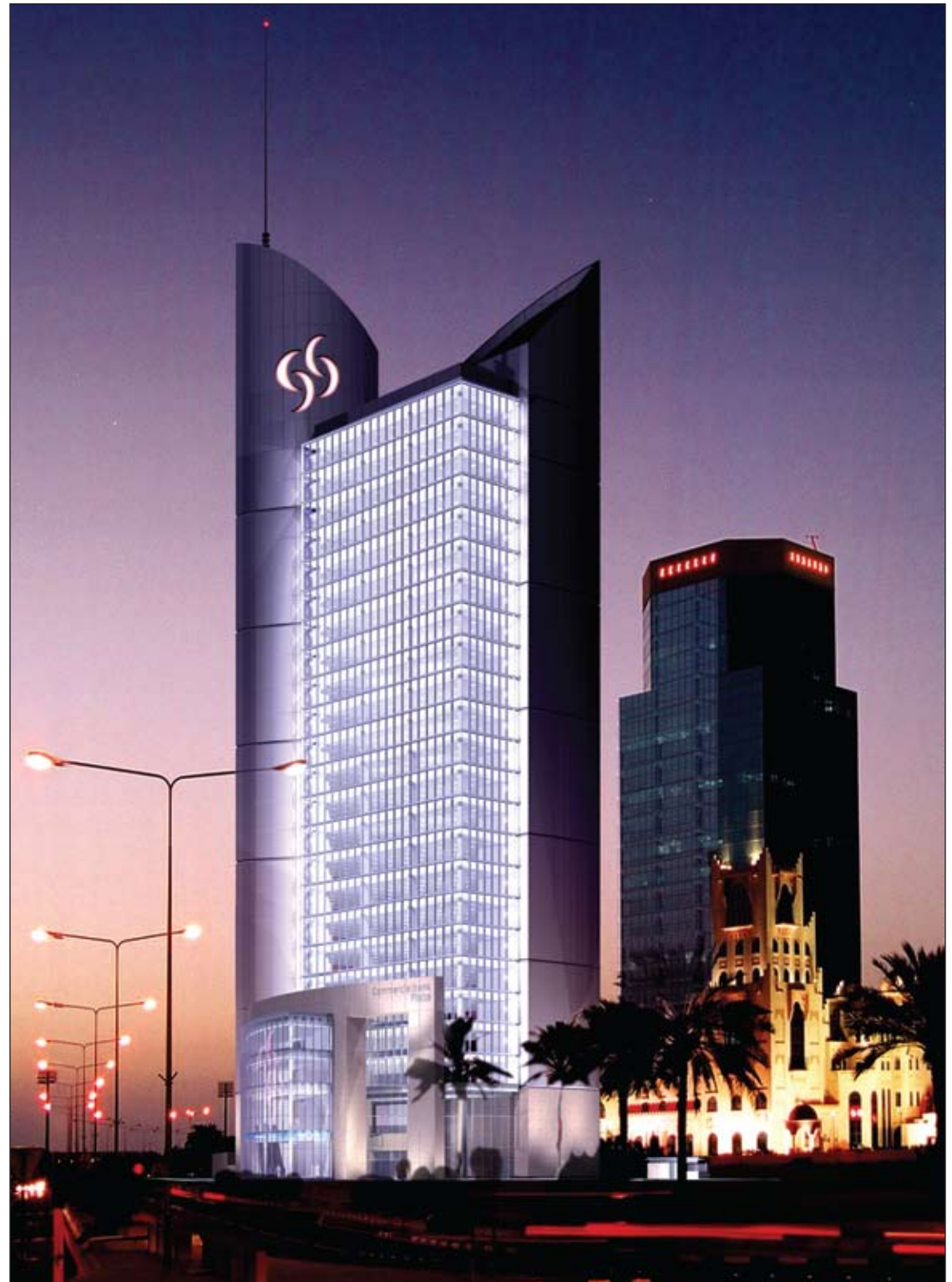
Commercialbank of Qatar's Doha headquarters
