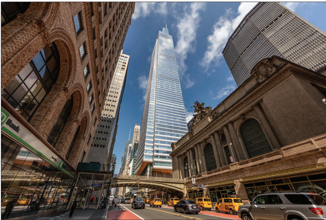
Standing 1,401 feet tall and totaling 1.7 million square feet, One Vanderbilt offers an unparalleled package of amenities, innovative office design, technology offerings, best-in-class sustainability practices and a prime location at the doorstep of Grand Central Terminal. The iconic tower is the tallest office tower in Midtown Manhattan.
