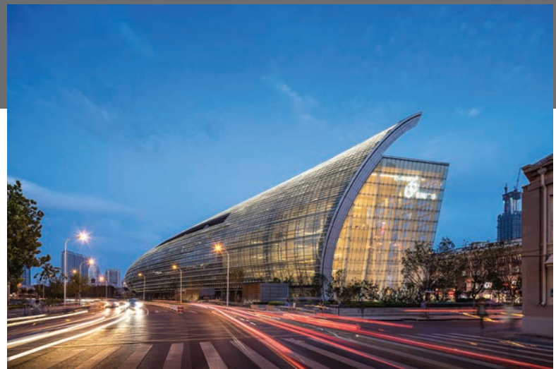
Riverside 66 in Tianjin, China
