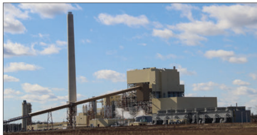
AEP's John W. Turk Power Plant near Fulton, Arkansas (above). The 600-megawatt Turk Plant is the first and only ultra-supercritical generating unit built in the U.S. Turk Plant generates electricity more efficiently at higher temperatures, requires less coal and produces fewer emissions to generate the same amount of power as other existing coal-fueled power plants. AEP 765-kilovolt (kV) transmission tower in Virginia (lower left). AEP built the first 765-kV (EHV) extra-high-voltage transmission lines in the United States and operates more EHV transmission lines than all other U.S. utilities combined.
