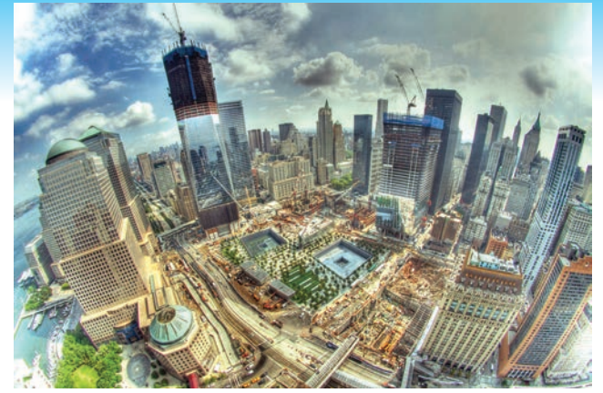
AECOM is deeply involved in the development of the new World Trade Center.
