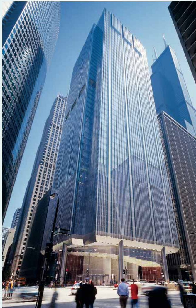
EMCOR's construction services helped build 111 South Wacker Drive, Chicago.
